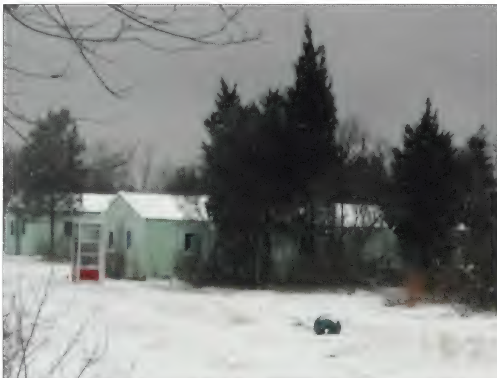
Figure 3.63. View looking northwest at the Ready Barracks, NIKÉ radar site. Pedestrian-scale lights line both walks from the control areas to the Ready Barracks. The lights are in good to fair condition with the exception of one light pole which is knocked over (Olmsted Center, January 2009).
